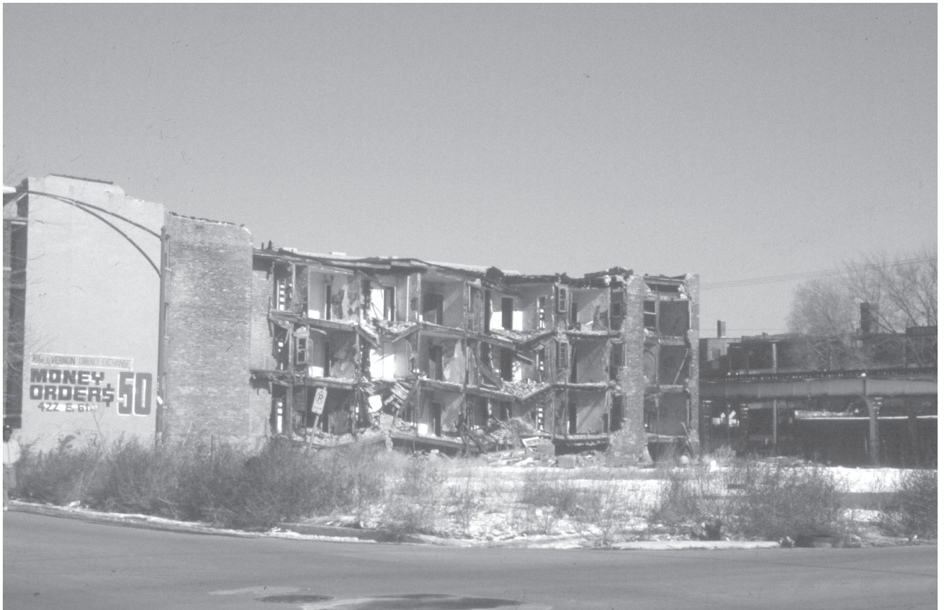
Crumbling buildings and urban desertification on Chicago's South Side
