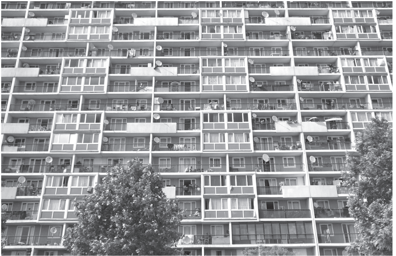
A typical building (called a "barre") in the estate of Les Quatre Mille
