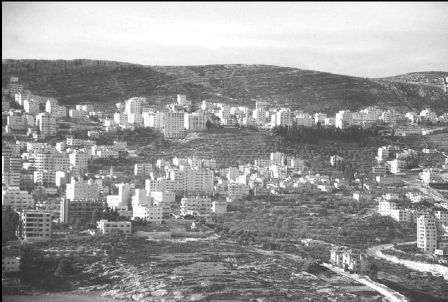
4. Nablus - Palästina: That dispersion is also possible with the typology of the high rise shows the example of the city of Nablus. In the western quarter Rafidiah limestone-towers grow in the terraces of the former olive gardens. In principle they are bloated single-family homes since they are normally built and used by large families. The capital usually comes from family members who have emigrated. The conversion of limestone into real-estate capital is economically sound and follows an unspoken rule of the conflict in the Middle East: "Who builds first, wins"
